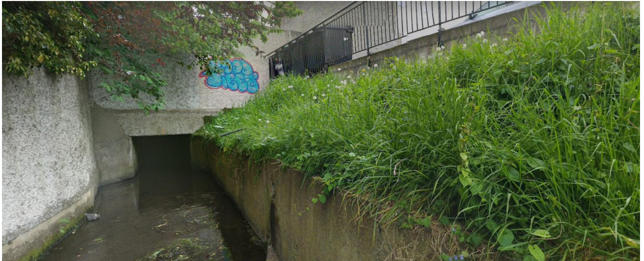
Existing culvert at location of proposed Kimmage 02 walkway
